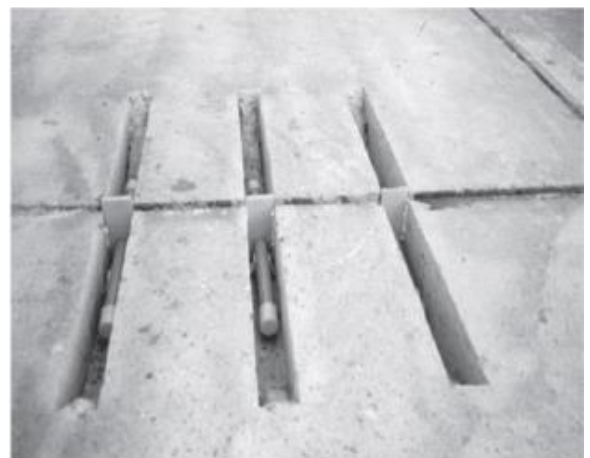
Placement of Dowel Bars
