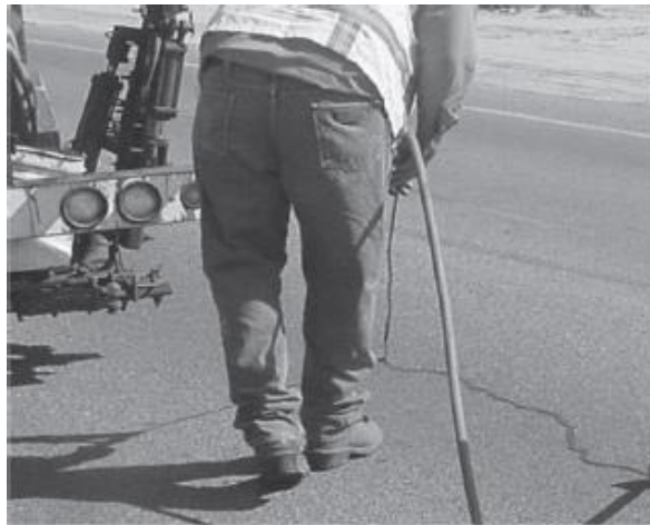
Crack Sealing
