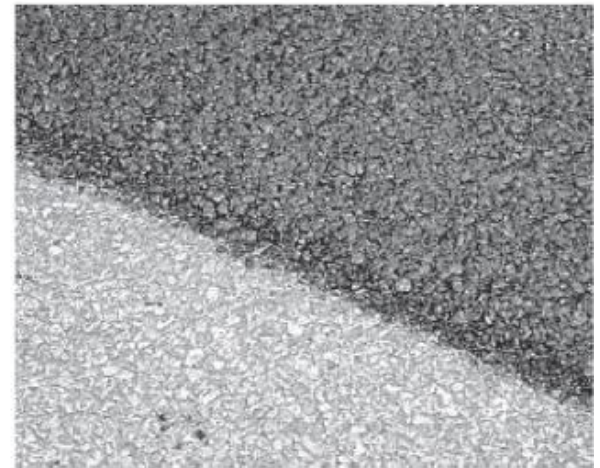
Thin HMA Overlay
