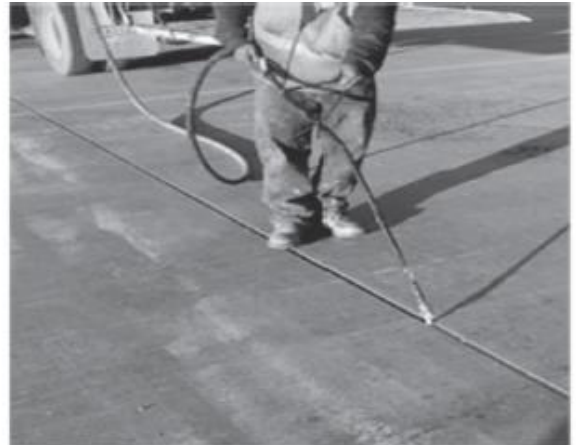
Joint Sealing
