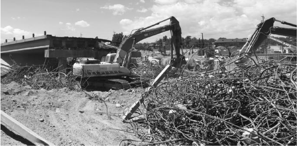
Figure 22 Steel Bar Removal from an Interstate Pavement
